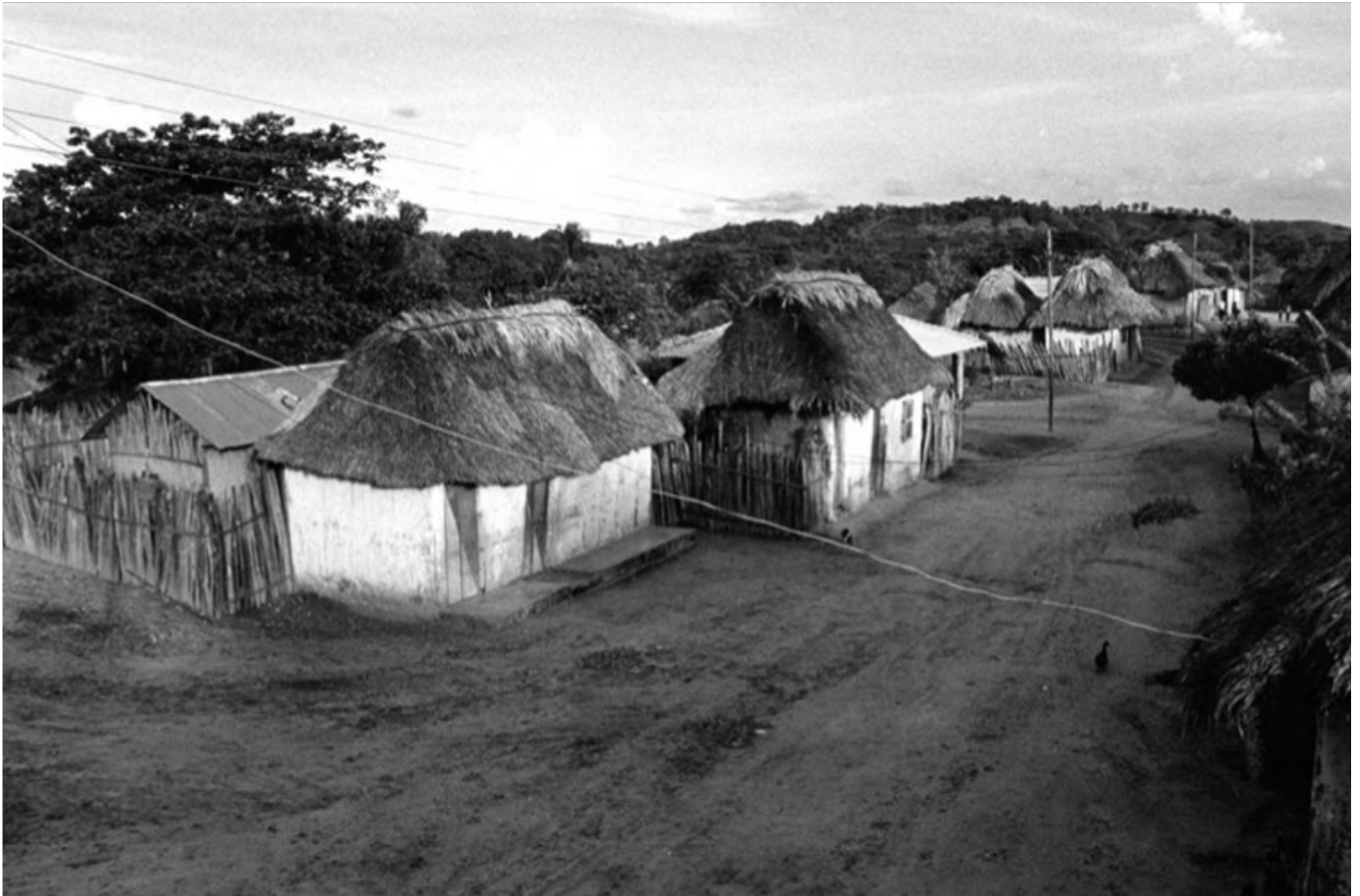
Electricity cables hanging between houses, San Basilio de Palenque, 1976
