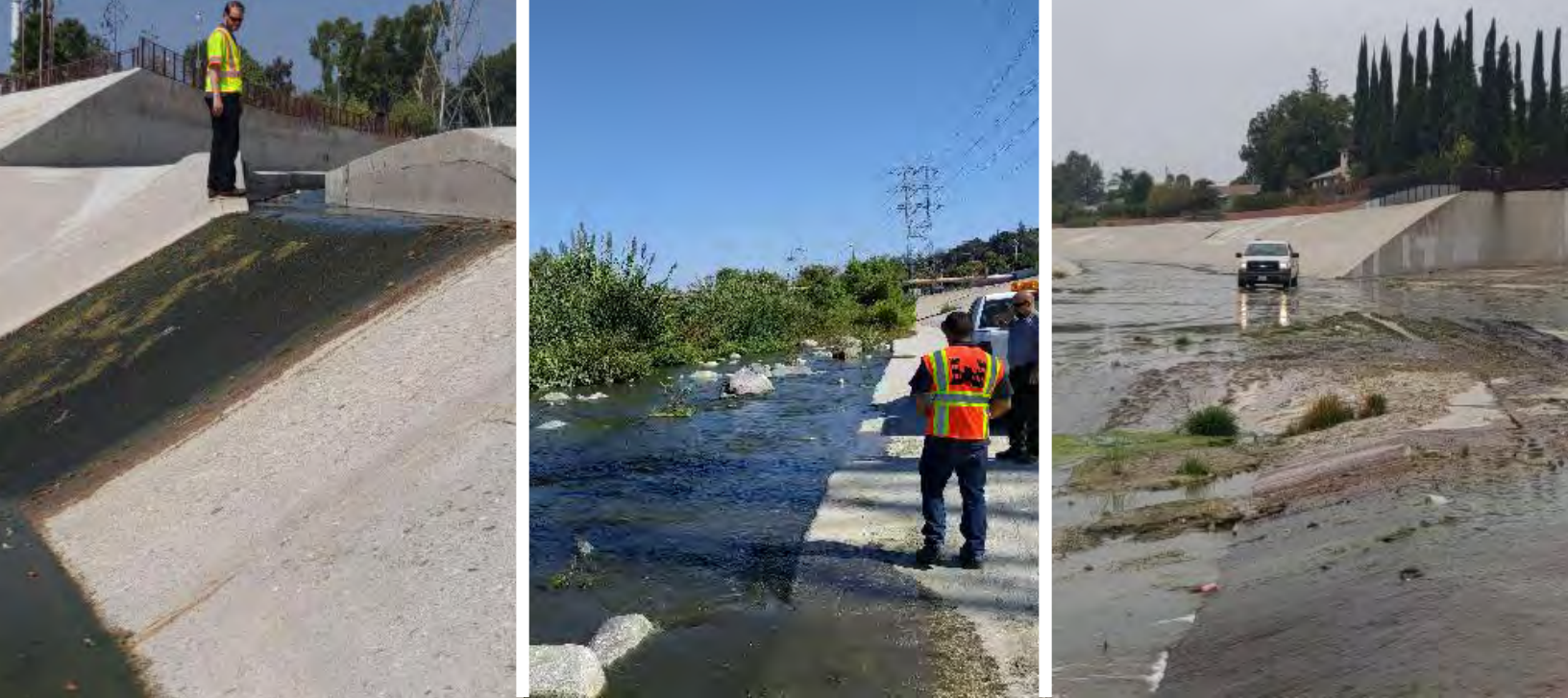
Figure 370. Outfall, soft bottom vegetation, river bottom inspection. Source: Geosyntec, 2018.
