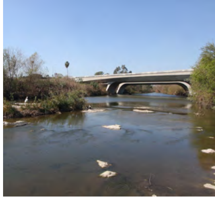
RIVER MILE 43: SEPULVEDA BASIN
