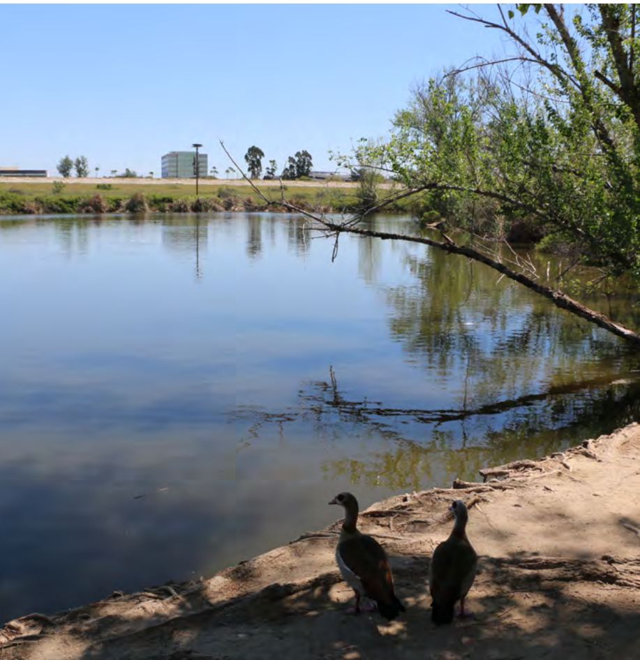
Figure 60. Sepulveda Basin's roughly 17,000 acre feet of storage provides significant flood risk management to downstream reaches. Source: OLIN, 2018.
