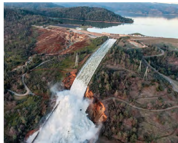
Figure 288. Oroville Dam. Source: Cal OES, Oroville Spillway, 2017.
